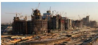
Wide construction site
