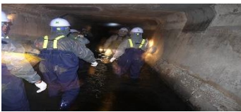
Sewer work site
